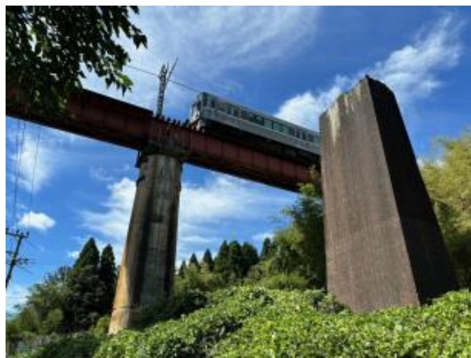
旧高屋川橋梁
